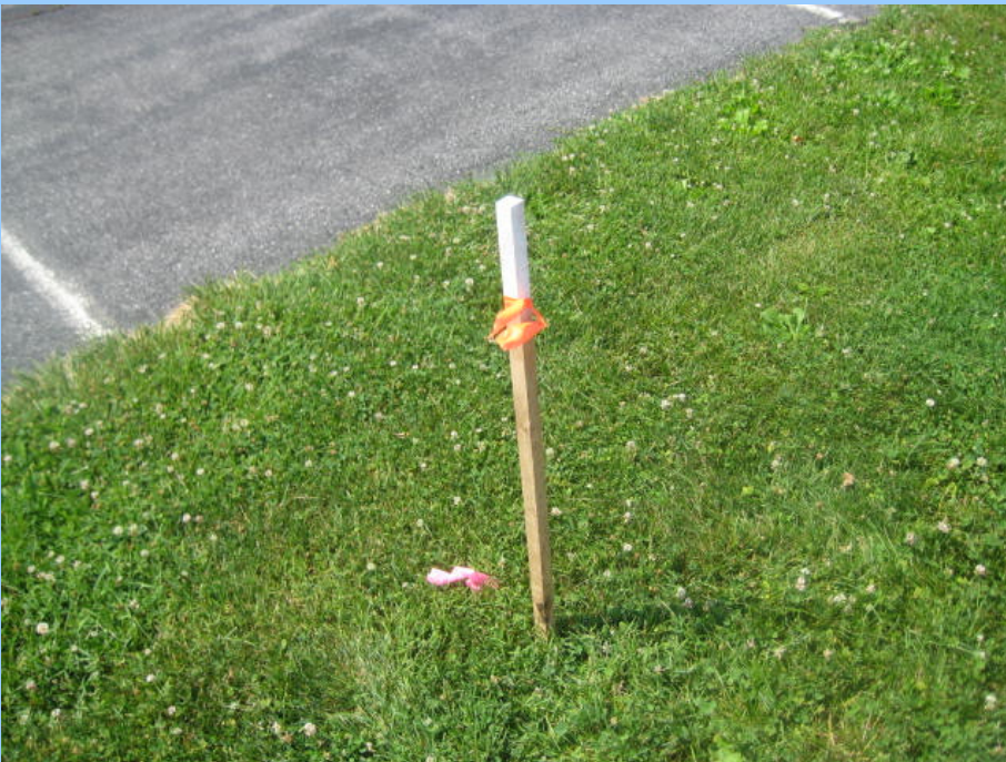
Excavating Stakes were placed!
